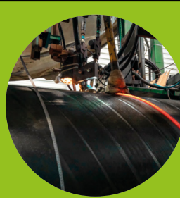
Solda Externa - SAW
